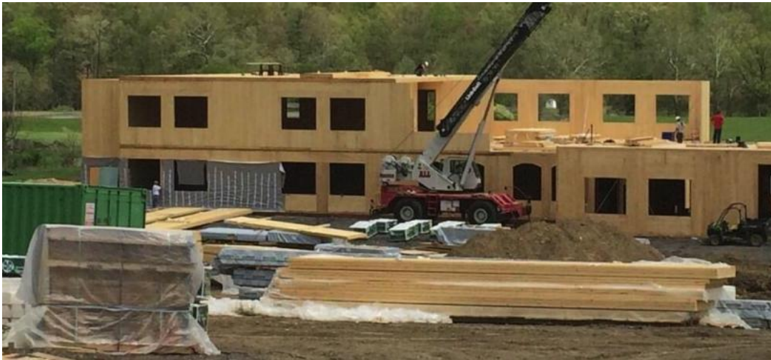
Franklin Elementary School Franklin, WV 45,200 sf 2-story Elementary School 2.5 months to erect CLT
