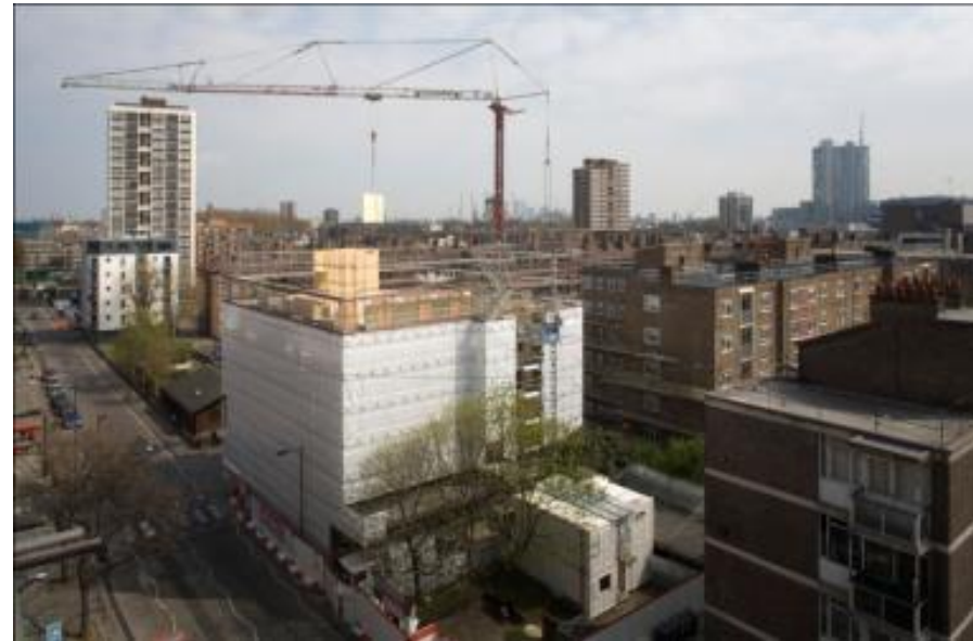
Murray Grove, London, UK 8 stories of CLT over 1 story concrete podium 8 stories built in 27 days (~1/2 the time of precast concrete)
