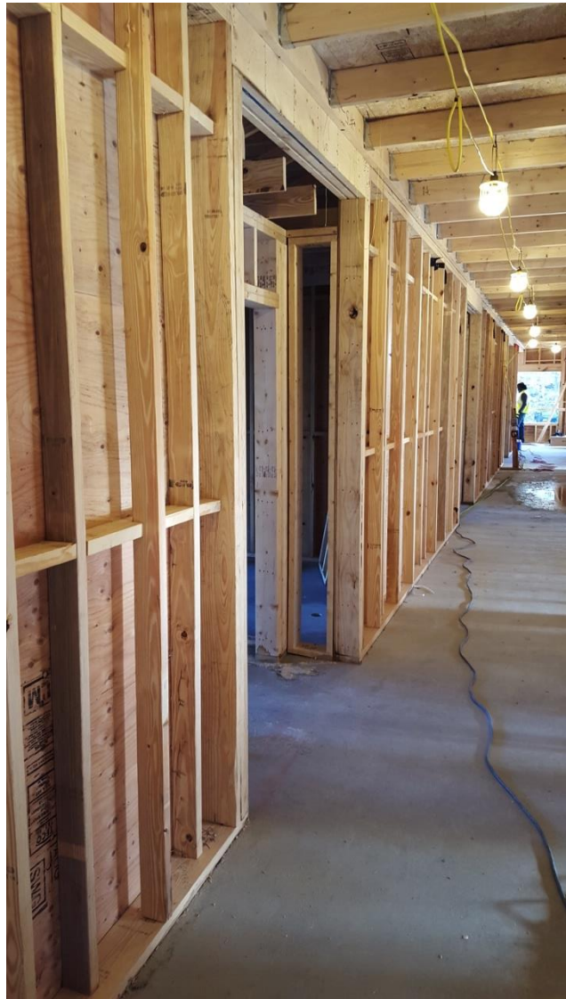
Light Wood-Frame Photo: WoodWorks
