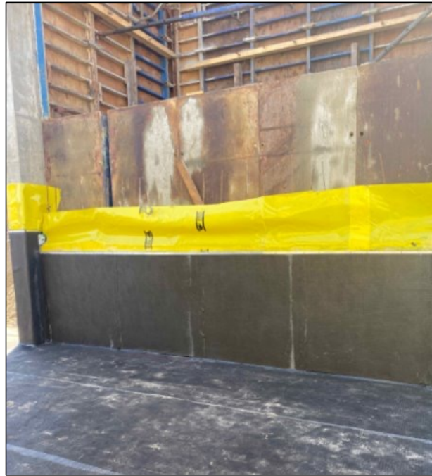
Below-grade waterproofing - Site observation
