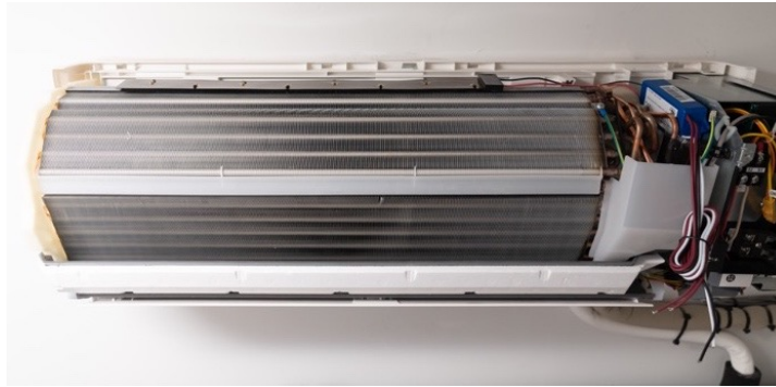
DUCTLESS MINI-SPLIT MOUNTED
