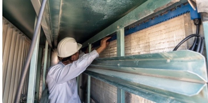
COOLING COIL MOUNTED
